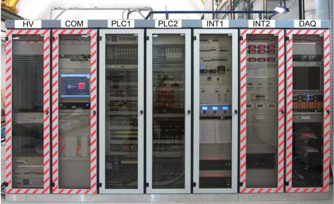
FIG. 62: The seven standard 19 racks containing the ArDM (CERN RE18) control system (COM, PLC1, PLC2, INT1 and INT2 rack), the high voltage supply of the PMTs (HV rack) and the data acquisition system (DAQ rack). The system was built in Collaboration with the CERN/PH-DT group.
